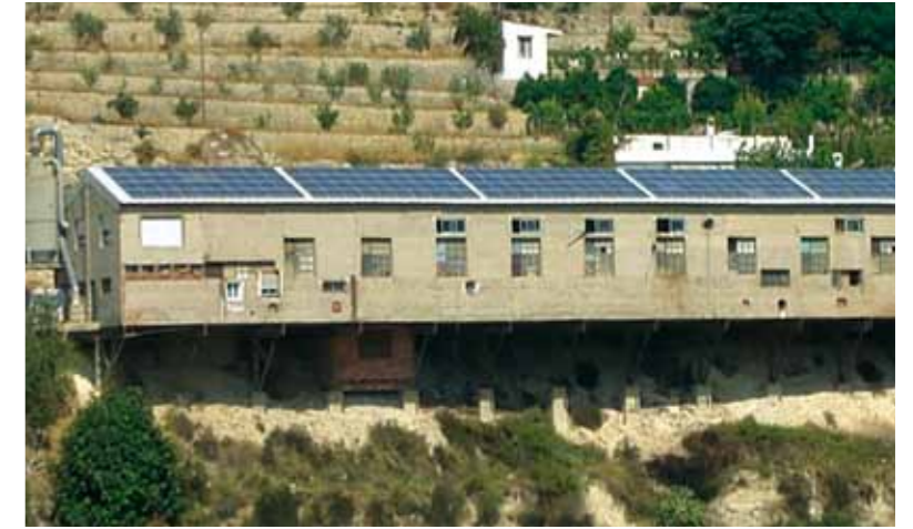
36,8 kWp in Jijona (Alicante) 210 panels, 290 m 2 Annual production 49.026 kWh
