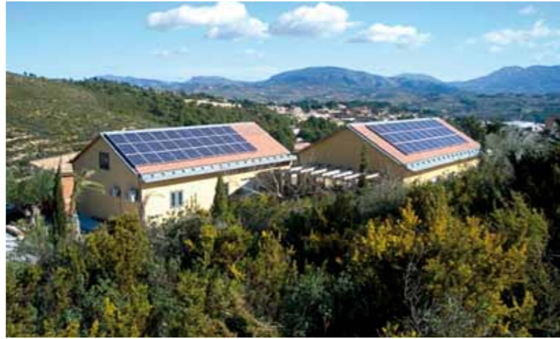
10 kW in Cocentaina (Alicante) 66 panels, 90 m 2 Annual production 16.414 kWh
