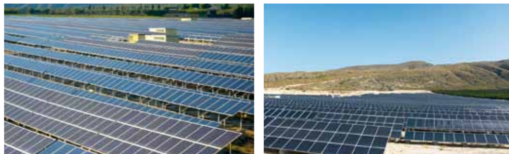
The photovoltaic panels are placed in their optimum inclination and orientation to maximize their performance.
