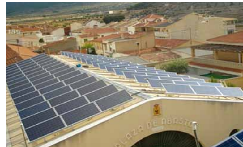
20 kWp City Hall in La Romana (Alicante) 120 panels, 160 m 2 Annual production 30.095 kWh
