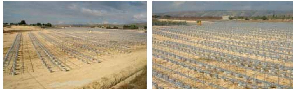
Clearing the land (around 70.000 m 2 ) and setting the metal structure for the panels.
